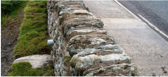
New drainage gully for standing water on bend
