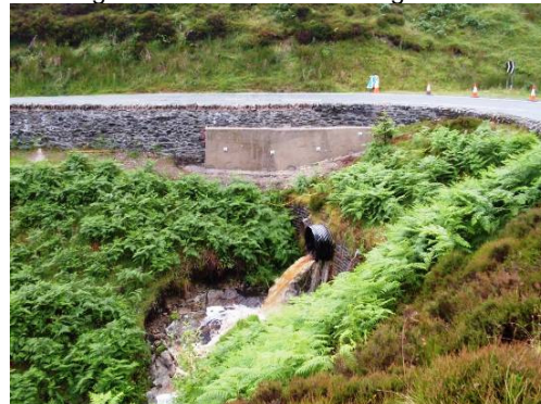
Anchored reinforced concrete buttress (prior to cladding)
