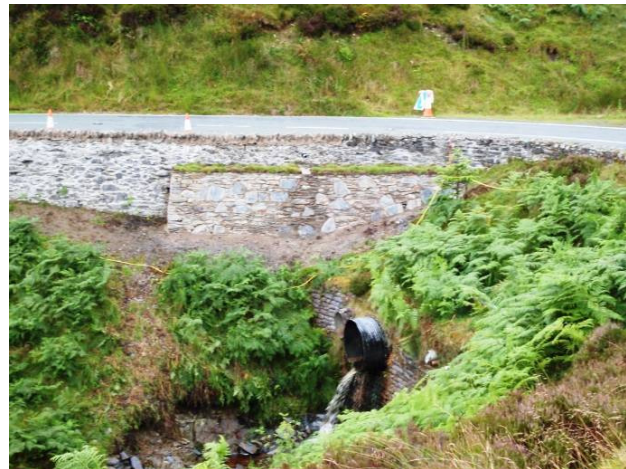
Concrete buttress clad in local stone to tie into existing wall
