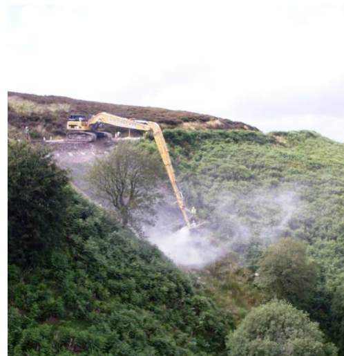
Long reach excavator installing soil nails
