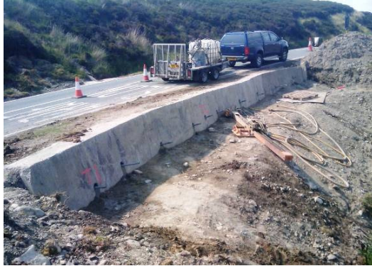
Extended and anchored top beam
